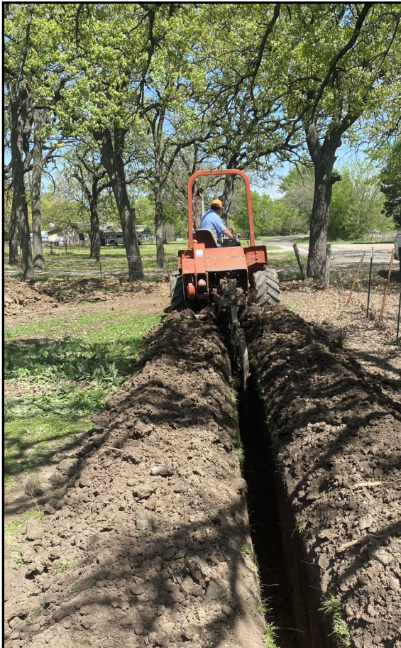
Pic 1: Trenching for water lines
