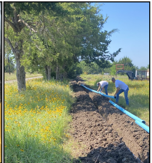
Pic 3: Installing water new water lines
