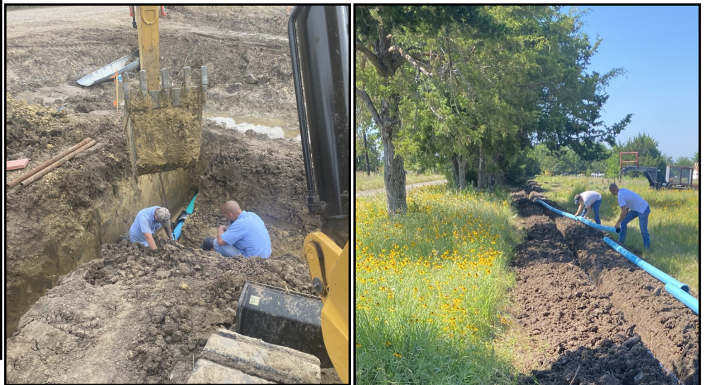
Pic 2: Installing a fire hydrant
