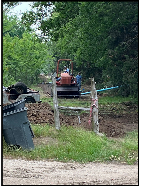
Picture on the Left: Installing the new 8" water line on Streetman Rd.
