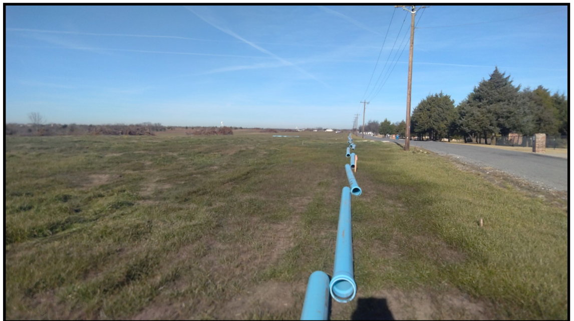
Picture on the Left: Installing new 8" line for Landon Estate
