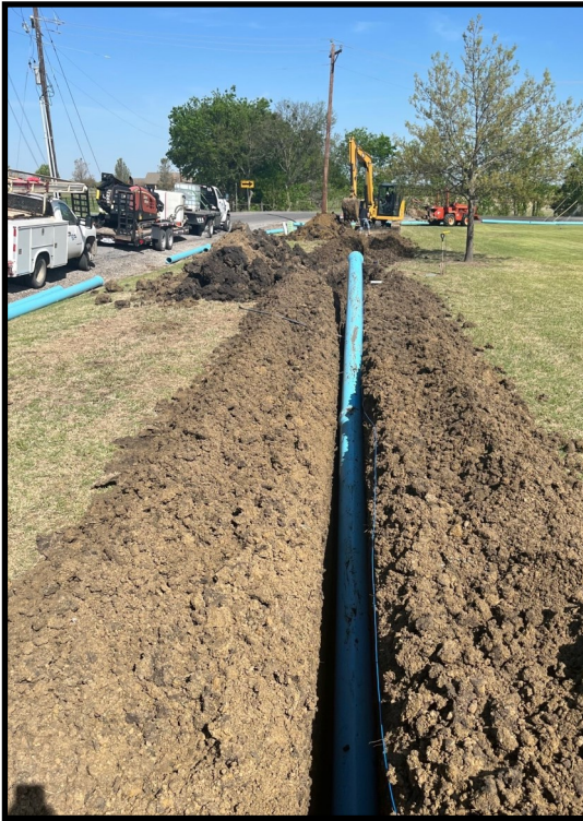
Picture on the Left: Installing the new 8" water line on Streetman Rd.
